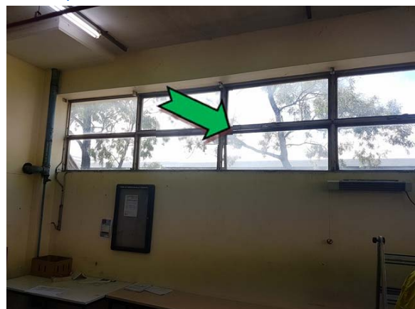
Photo 6. Interior, ground level, throughout, window frames – non asbestos-containing caulking.
