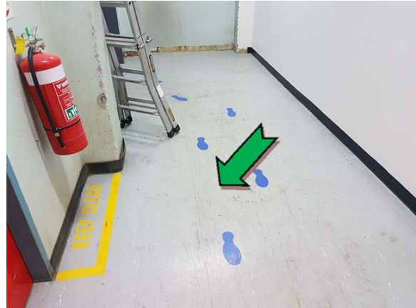
Photo 2. Interior, level 1, throughout, floor – non asbestos-containing vinyl floor sheeting.
