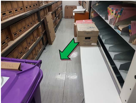
Photo 3. Interior, level 1, throughout, floor – non asbestos-containing vinyl floor sheeting.
